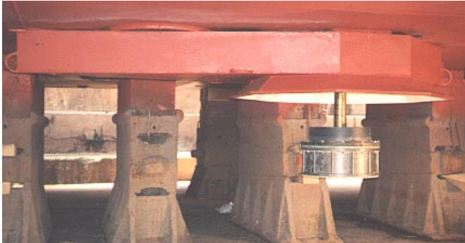
Figure 1 The tear-drop shaped bubble deflector shield installed on the hull of Discovery with the inner bell-shape transducer shield. The transducer itself was not yet in its operating position when its face would be just within the hull.
